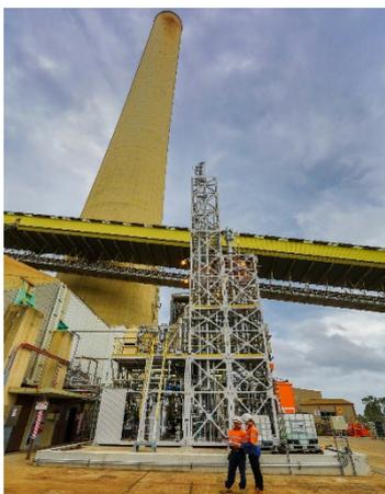
Figure 1: The PICA (PCC IHI CSIRO AGL) 150 tonnes CO<sub>2</sub>/annum carbon capture pilot plant located at the AGL Loy Yang Power Station, Victoria, Australia.
