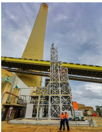
Figure 1: The PICA (PCC IHI CSIRO AGL) 150 tonnes CO 2 /annum carbon capture pilot plant located at the AGL Loy Yang Power Station, Victoria, Australia.
