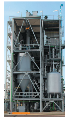
TUF fixed bed gasifier test facility
