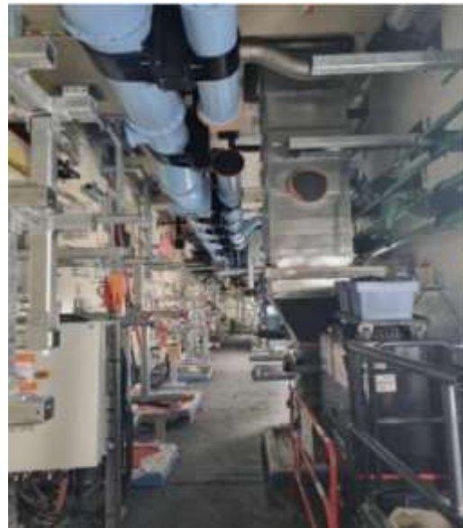
Implementation of Equipment @ level -3
