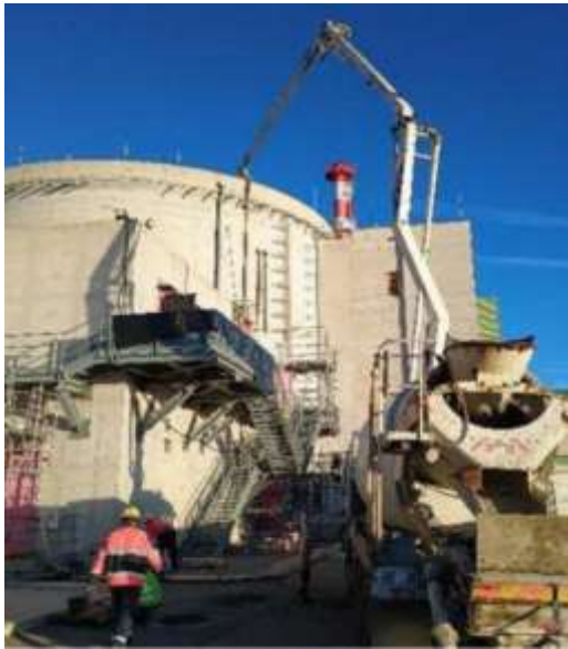
Concrete pouring in Safeguard building
