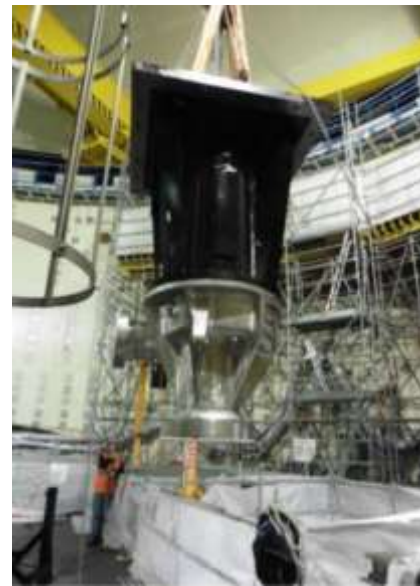
Primary pump assembly: support, volute
