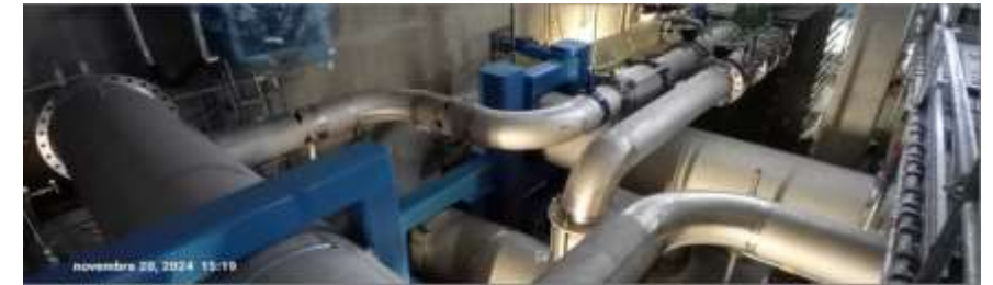
Installation of supports and pipes in the Cooling Circuit Building
